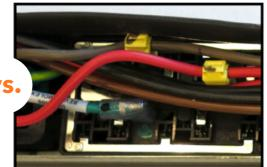
Quick to overheat and fail Hand-work mechanical terminations.
